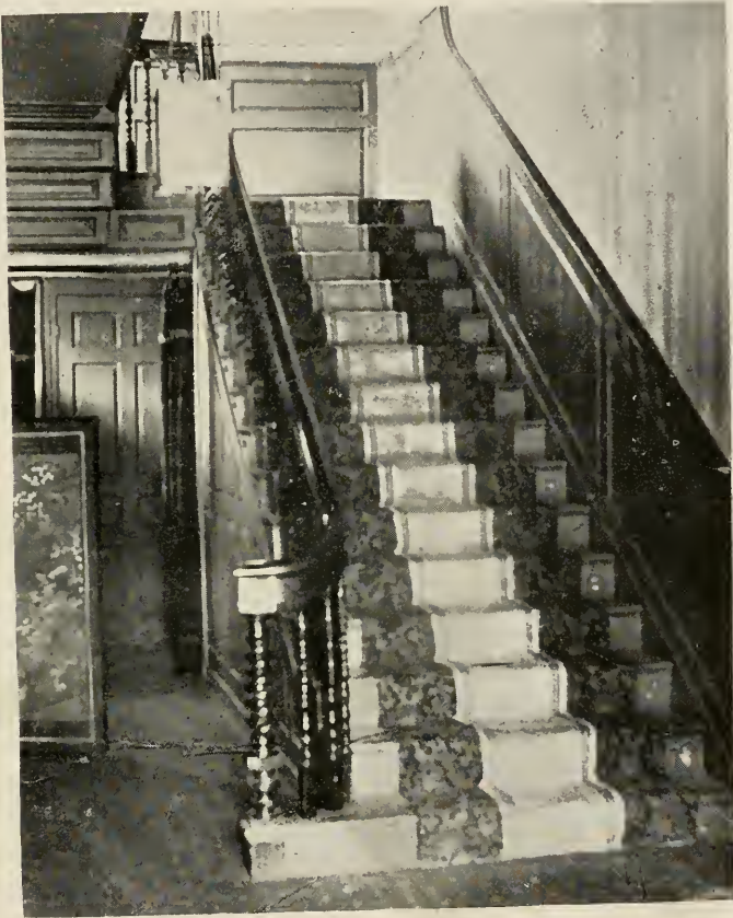
HALL AND STAIRCASE, DALTON HOUSE.
